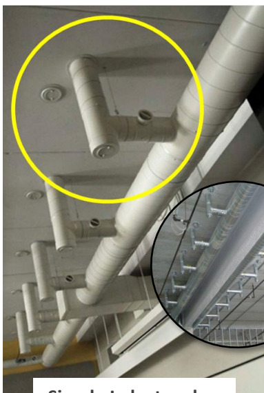
Simple L-duct makes the connection
