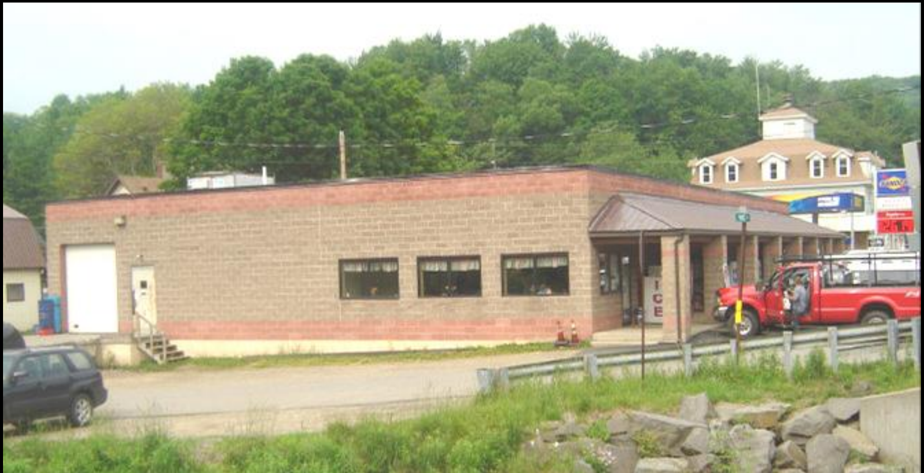
Don Reed's 6800 square foot grocery store, in Genesee, PA. A few miles south of the NY state line. Erected 1994, using 10" CICMU's. Climate zone 6.
