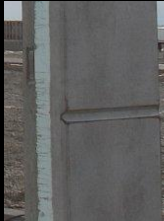
Concrete sandwich panel
