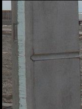
Concrete sandwich panel
