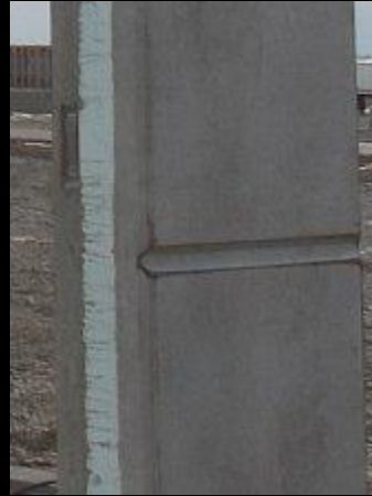
Concrete sandwich panel
