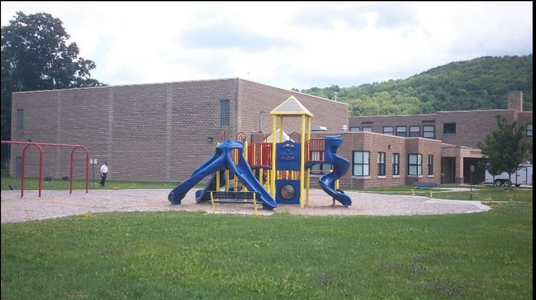
CICMU school addition and gymnasium.
