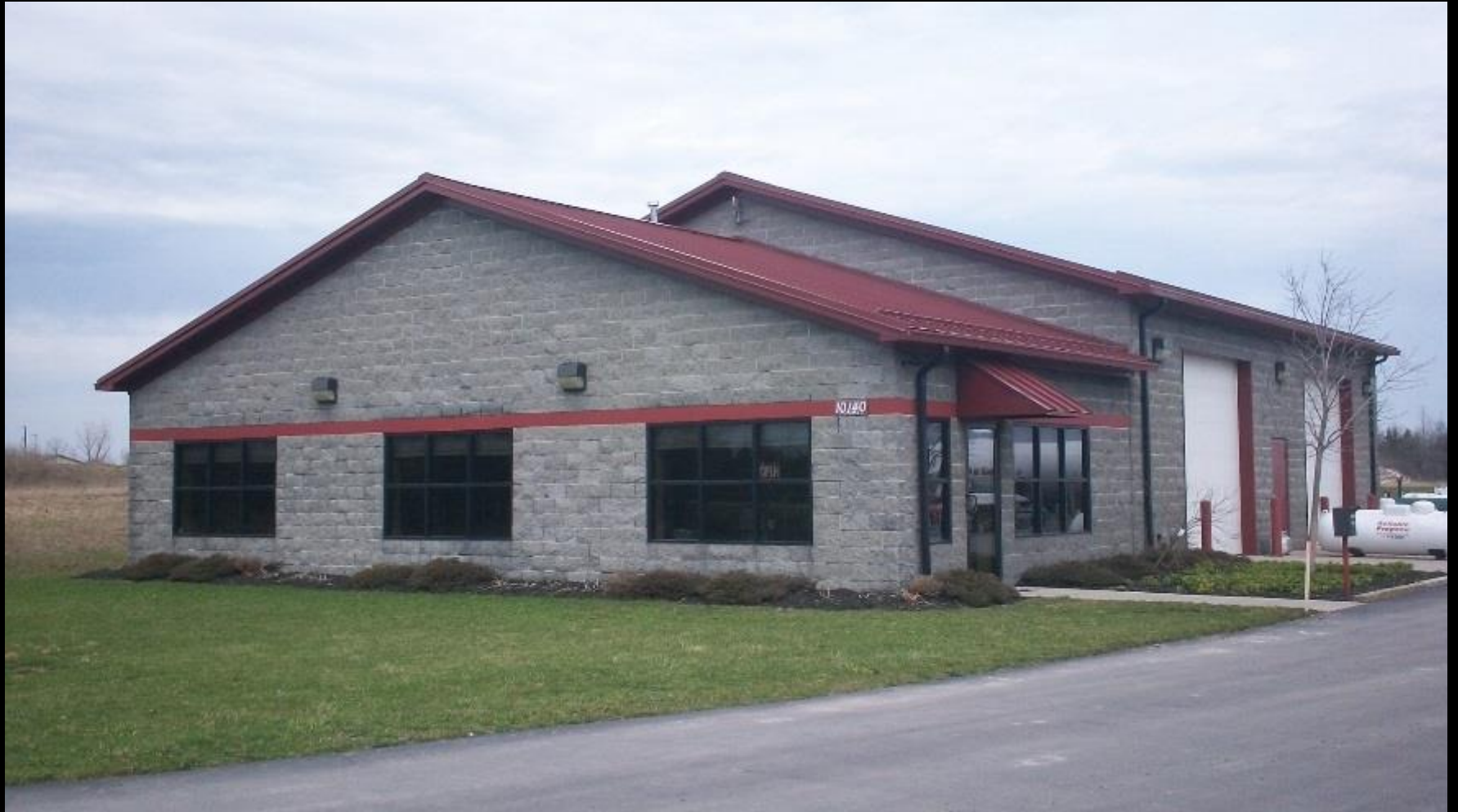
CICMU Small office with garage.
